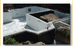
A Quad-Lock finished basement can be built in about 60% of the time of a traditional finished basement. Although the concrete costs are similar, elimination of secondary framing and insulation steps save both time and money.
