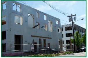
After having used other ICF systems in the past, Northern Hills chose Quad-Lock specifically for its ease of use and the incorporation of the Quad-Deck Green Roof application. The two buildings, totaling over twelve thousand square feet of living area have walls thirty-five feet high finished with stucco exterior. Quad-Lock ICFs were also used for the interior firewalls. The creation of this superior building envelope allows for even greater energy
