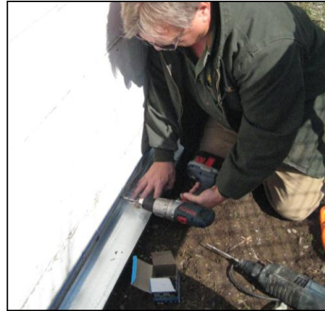
Figure 8: Fastening R-ETRO Plus Track
