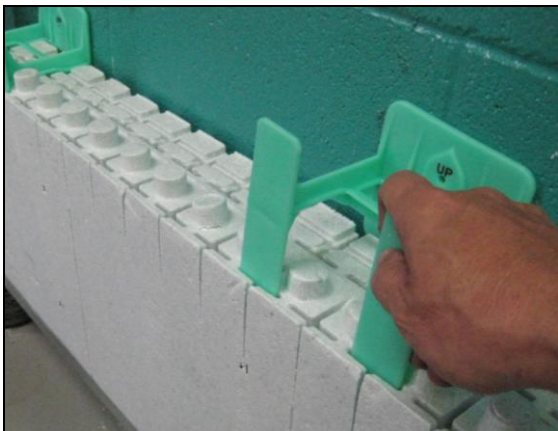
Figure 10: Place R-ETRO Plus Tie in Plus Panel
