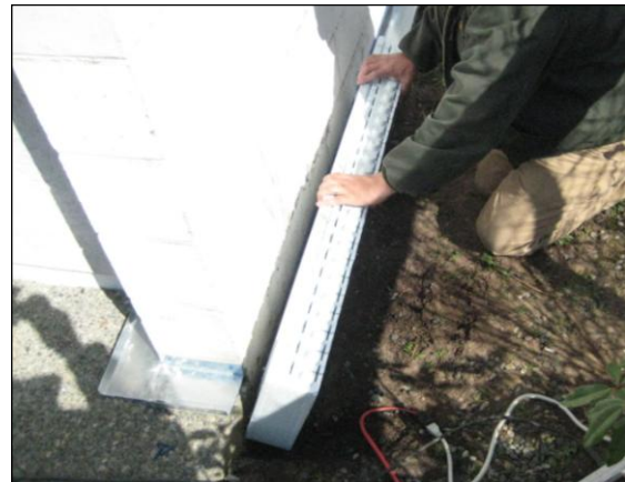
Figure 9: Place Plus Panel in R-ETRO Track
