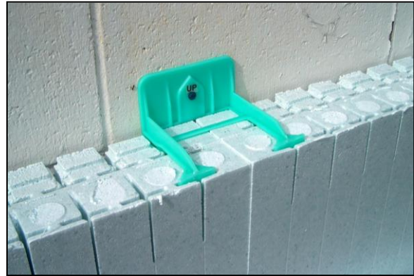
Figure 21: R-ETRO Plus Top Tie Installation
