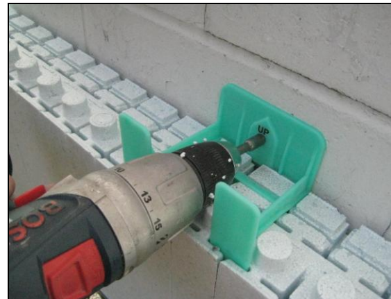
Figure 11: Fasten Ties to Wall
