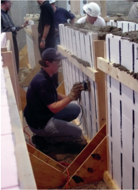
Figure 9. Concrete consolidation using an orbital sander. (IMG13341)
