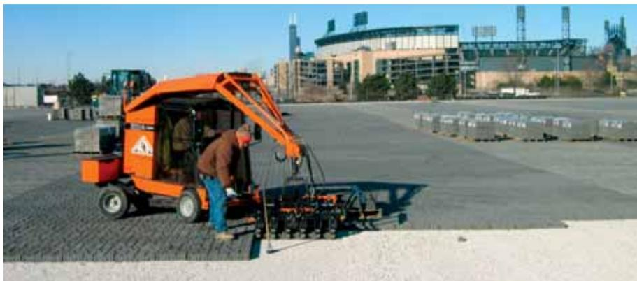
Unilock's Eco-optiloc precast permeable concrete pavers were used to create the largest permeable parking lot on record at Chicago's U.S. Cellular Field. The park's drainage capacity is 1.15 million gallons—or 9.25 million 16-oz. sodas. Image courtesy of Rose Paving and Unilock.
