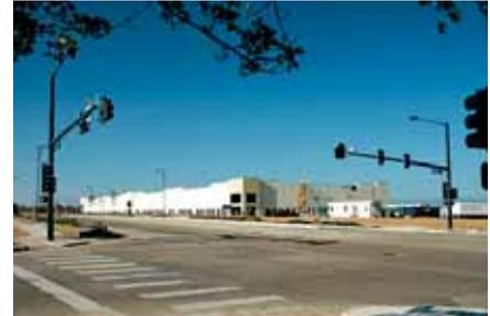
Tilt-up buildings at Enterprise Park, located at the site of the former Stapleton Airport, contain a large amount of recycled concrete aggregate in both foundations and tilt-up components. Images courtesy of ReCrete Materials, Inc.
