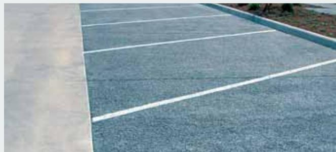
At the Prime Outlets, conventional concrete was used for traffic lanes, while pervious concrete was used for parking stalls. Image courtesy of Titan Virginia Ready Mix.
