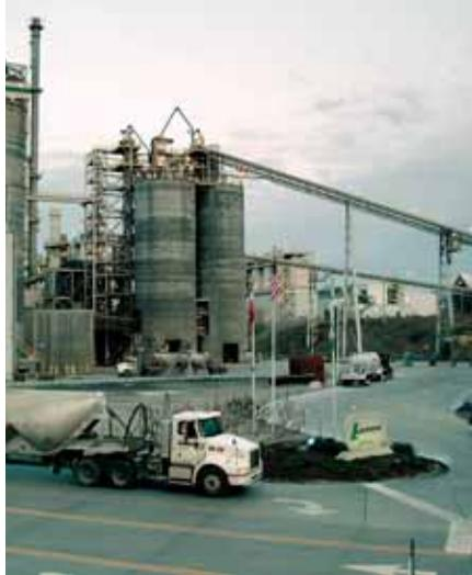
At Lafarge North America, Inc.'s Sugar Creek, Mo., cement plant, 33 percent of raw materials come from alternative sources like local utility bottom ash, boiler slag, foundry sands, iron mill scale and limestone fines. Image courtesy of Lafarge North America.
